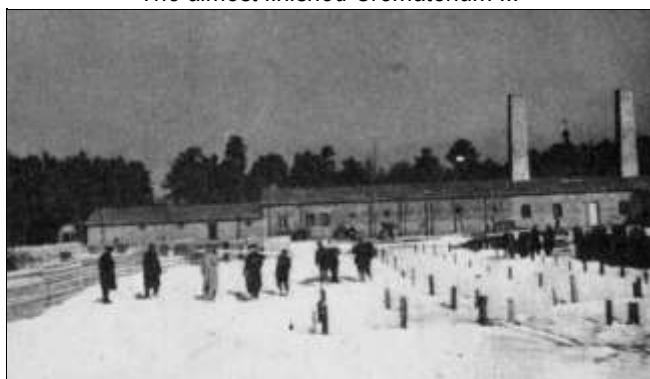
The finished Crematorium IV.
